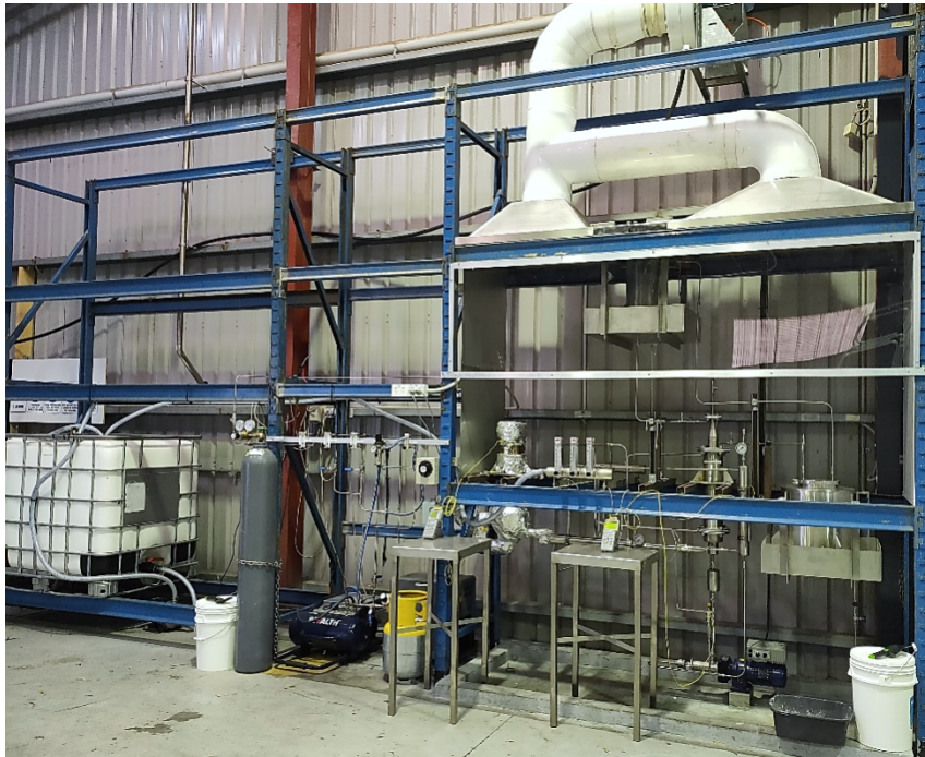
Figure 1: Alcore reactors for production of oleum
