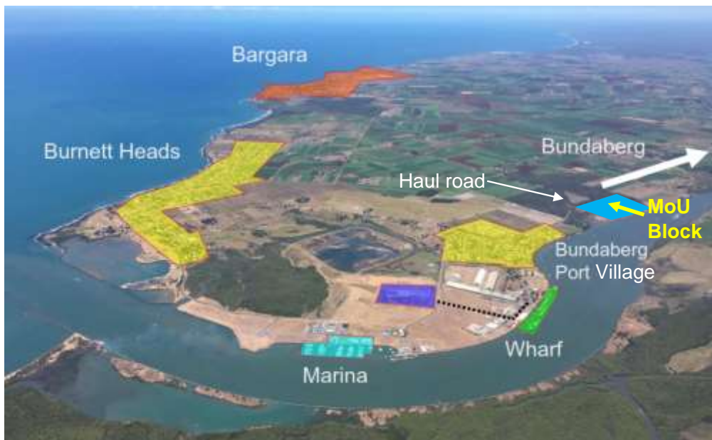
Figure 10: Location of the “MoU Block” (middle right) being assessed at the Port of Bundaberg
