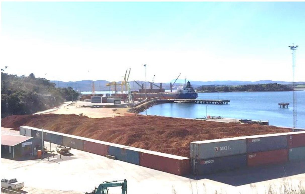
Figure 2: Bulk loading of 35,000 tonnes of bauxite from the port stockpiles (foreground) into the ship (in the background). The two cargoes are surrounded by old shipping containers used as windbreaks at Bell Bay export port, Tasmania
