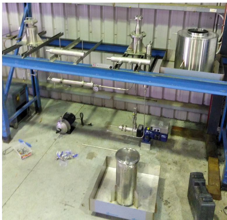
Figure 3: Pilot scale reactors being assembled in pilot plant facility
