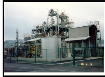
50,000 tpa Corethane Refinery mid 1980s US Military Base in Japan 1981-87 Corethane for gas turbines (Abrams M1 Tanks)
