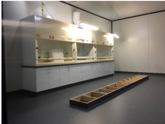
Floors are now sealed with hi-tech industrial vinyl (robust, anti-static & chemically stable). Kick-boards are the base for benches. All vinyl is turned-up the walls to seal the Core Lab.
