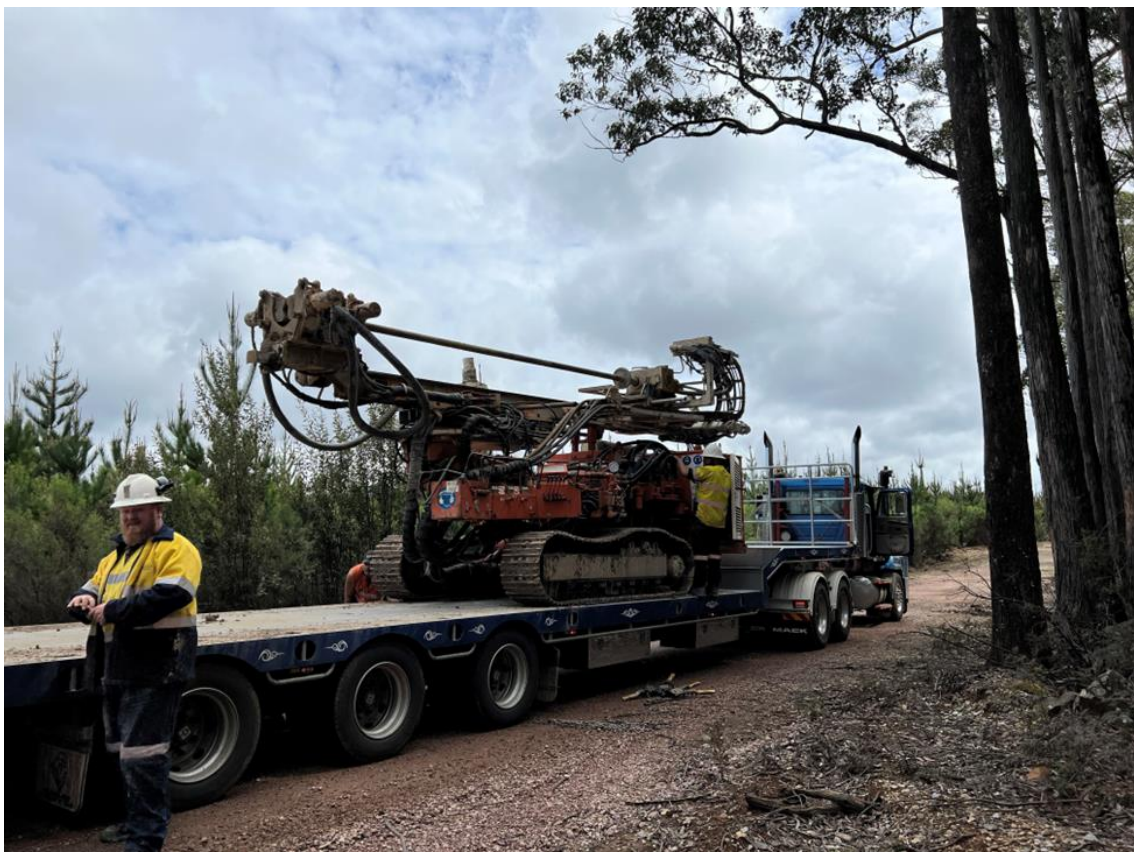
Figure 4: eDrill senior driller, Brodie Linger driving the eDrill RC drill rig off the low loader by remote controls
